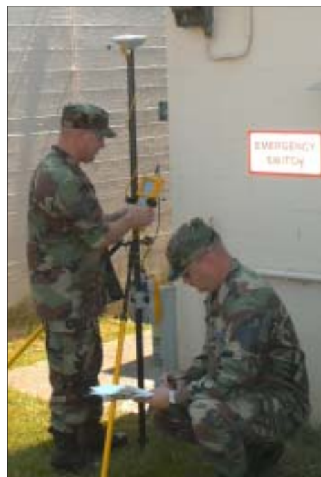
Tech. Sgt. Randy Sargent uses a Trimble GPS pedestal mounted unit to map copper telephone and fiber optics locations as Tech. Sgt. Michael Straley documents how much fiber was in use and the path the fiber took. Both are assigned to the 445th Communications Flight. (Courtesy photo)
